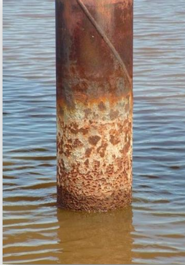
Coating Failure on Steel Pile
