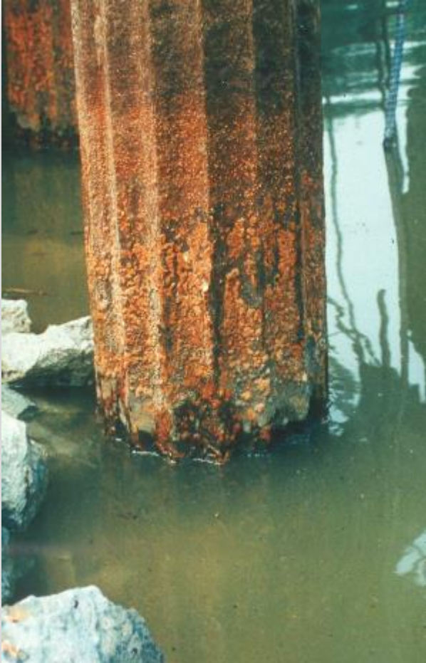
Uncoated Steel Pile
