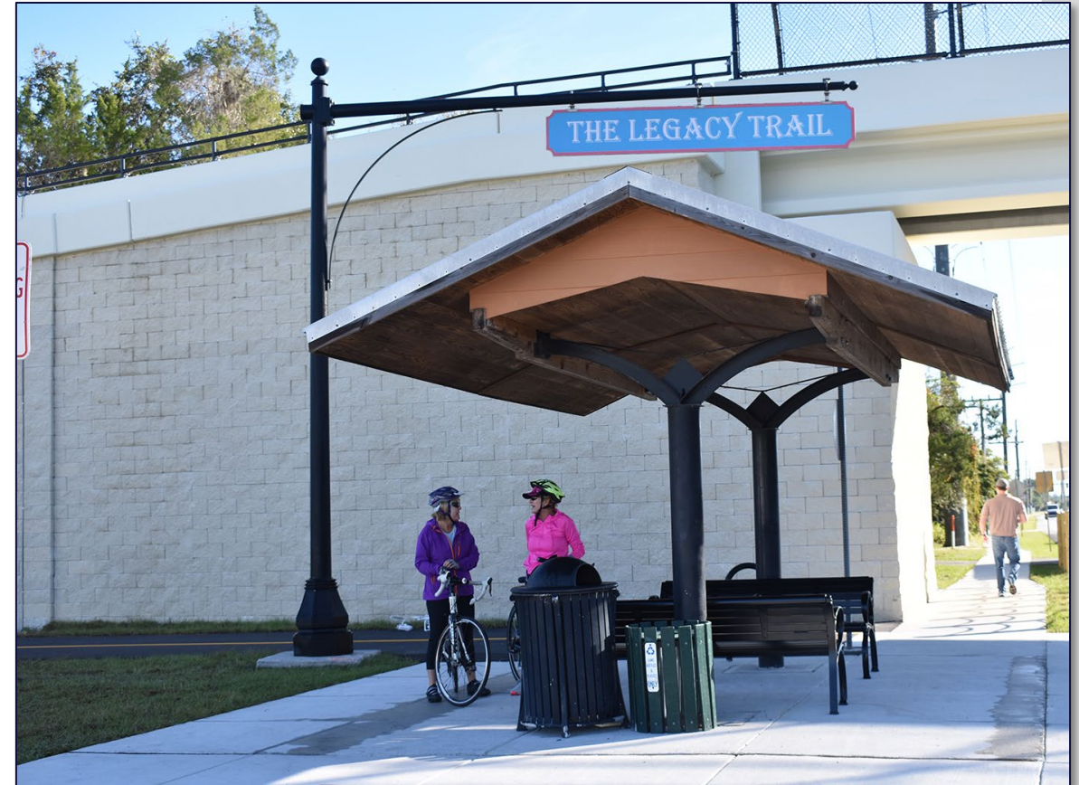
Legacy Trail Ped. Overpass at Laurel Rd. (LAP project) FDOT District One | Sarasota County FES Myakka Chapter Project of the Year
