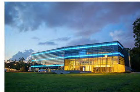
Structure Foundation Support
