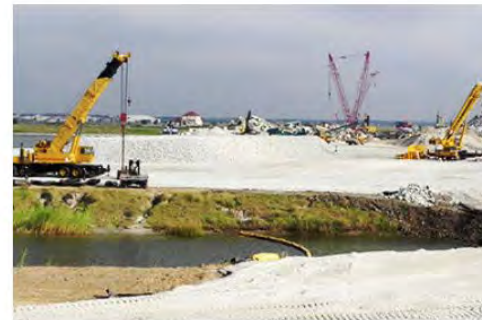
Marine Foundation Improvement
