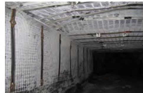
Underground Mining Support
