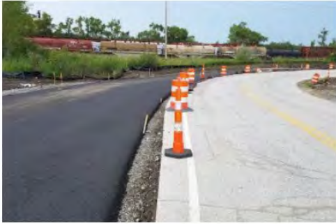
Roads, Pavements & Surfaces
