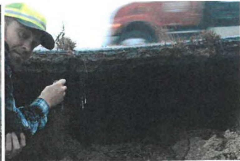
Figure 4.3.2-4—Bridging in Flexible Pavements (Photos courtesy of Minnesota DOT)
