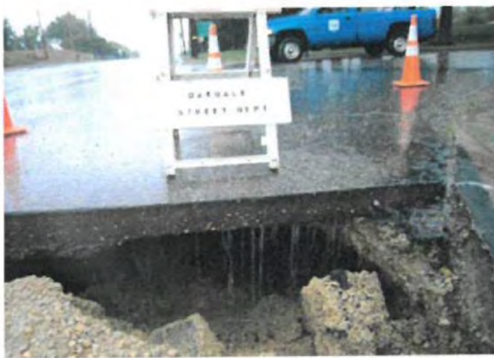
Figure 4.3.2-4—Bridging in Flexible Pavements (Photos courtesy of Minnesota DOT)
