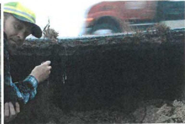
Figure 4.3.2-4—Bridging in Flexible Pavements
