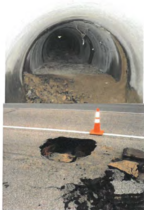
Figure 4.14.1-5—Severe Infiltration Through Joints in Concrete Pipe (Top). Surface Distress in Approach Roadway Caused by Loss of Backfill Due to Joint Infiltration. (Photos courtesy of Utah Department of Transportation (top) and Minnesota Department of transportation (bottom))
