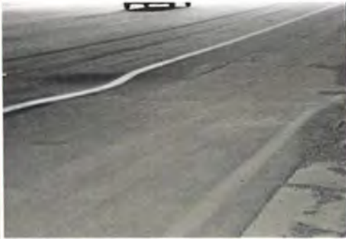
Courtesy of Minnesota Department of Transportation High-severity sags in roadway over culvert barrel.
