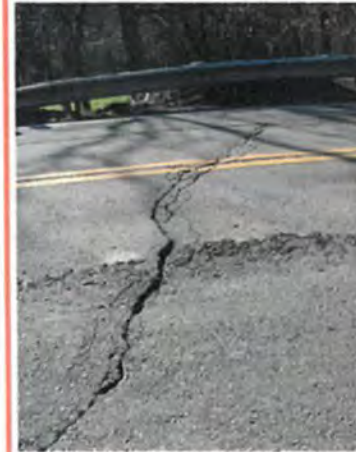
Courtesy of Minnesota Department of Transportation High-severity transverse cracks and high-severity sag over culvert barrel.
