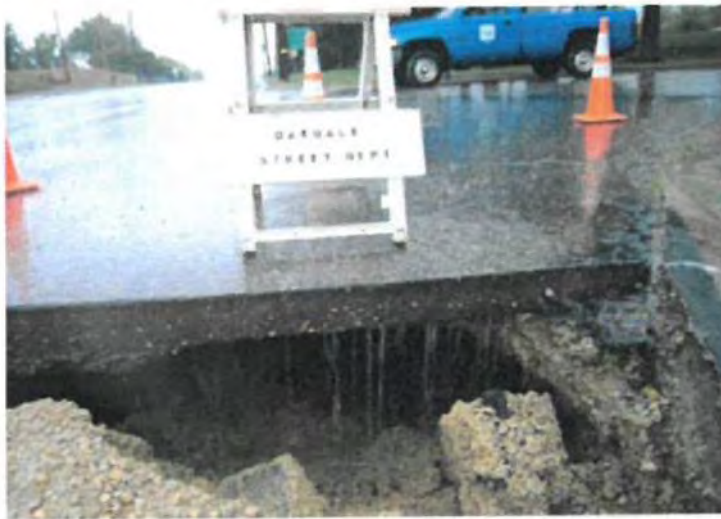
Figure 4.3.2-4—Bridging in Flexible Pavements
