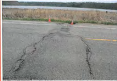
Courtesy of Minnesota Department of Transportation High-severity transverse cracks and high-severity sag over culvert barrel.
