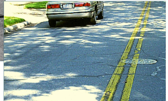
Slightly distressed surfaces - minor cracks, patches, etc.
