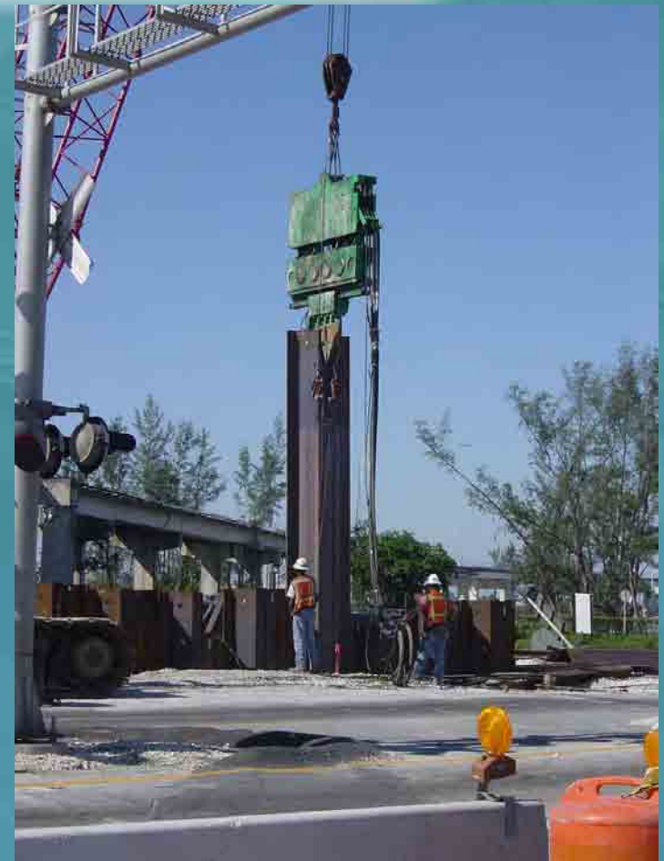
Sheet Pile Installation
