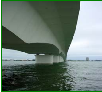
Ringling Bridge Across Sarasota Bay
