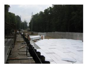
Geo-foam blocks were selected, and 13,000 cubic yards were trucked to the site from Miami in 41" x 49" x 194" sections. Designed to have a low density of 1.5 lbs/CF, these blocks strengthen the foundation of the bridge approach and reduce long-term settlement potential. The geo-foam block construction also limited the area of disturbance and therefore the environmental impacts. This was all done within a limited 100 day road closure.
