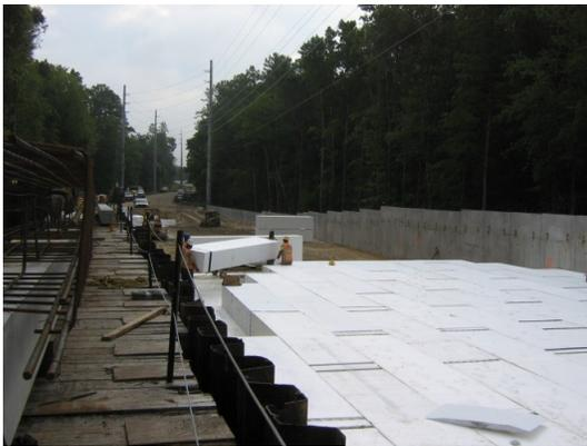
Geo-foam blocks were selected, and 13,000 cubic yards were trucked to the site from Miami in 41" x 49" x 194" sections. Designed to have a low density of 1.5 lbs/CF, these blocks strengthen the foundation of the bridge approach and reduce long-term settlement potential. The geo-foam block construction also limited the area of disturbance and therefore the environmental impacts. This was all done within a limited 100 day road closure.
